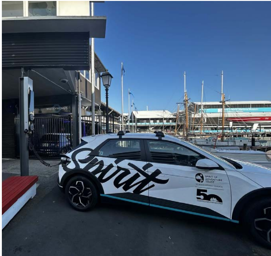
EV charging station
